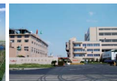
TBR Plant in Xiasha
